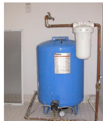
Figure 5. Example bladder pressure (blue) tank.
